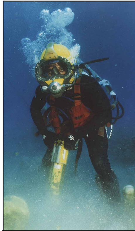
Figure 6-4. Underwater Construction Diving.
